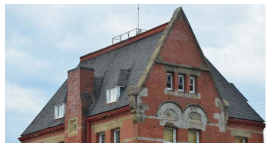
Figure 2: South east corner of Old Town Hall (Photo Credit: John Leroux)
